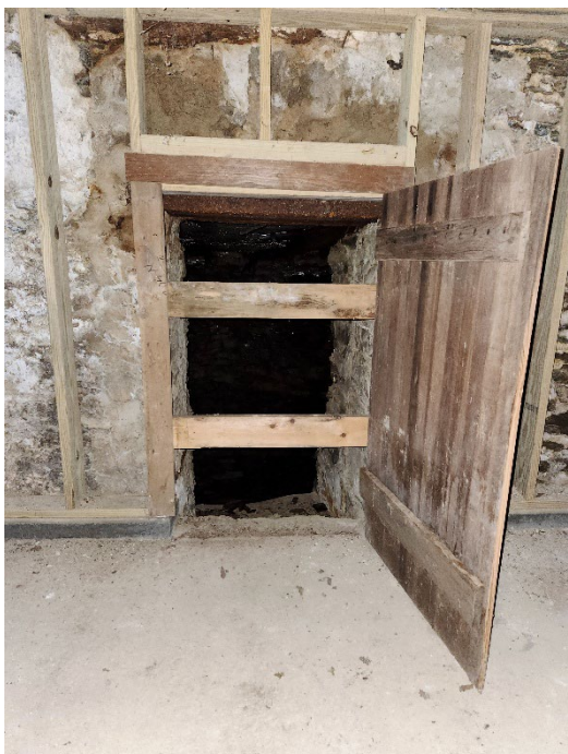
Figure 6: Illustration of an icehouse comprising a pit and frame enclosure.
