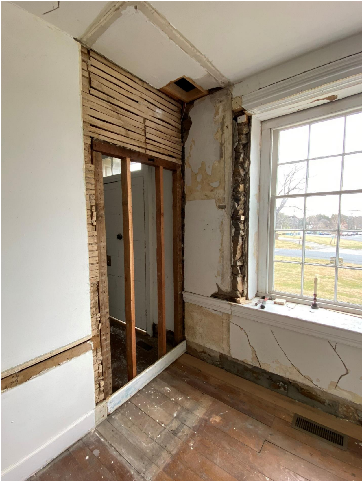
Front closet door opening infill "BEFORE"
