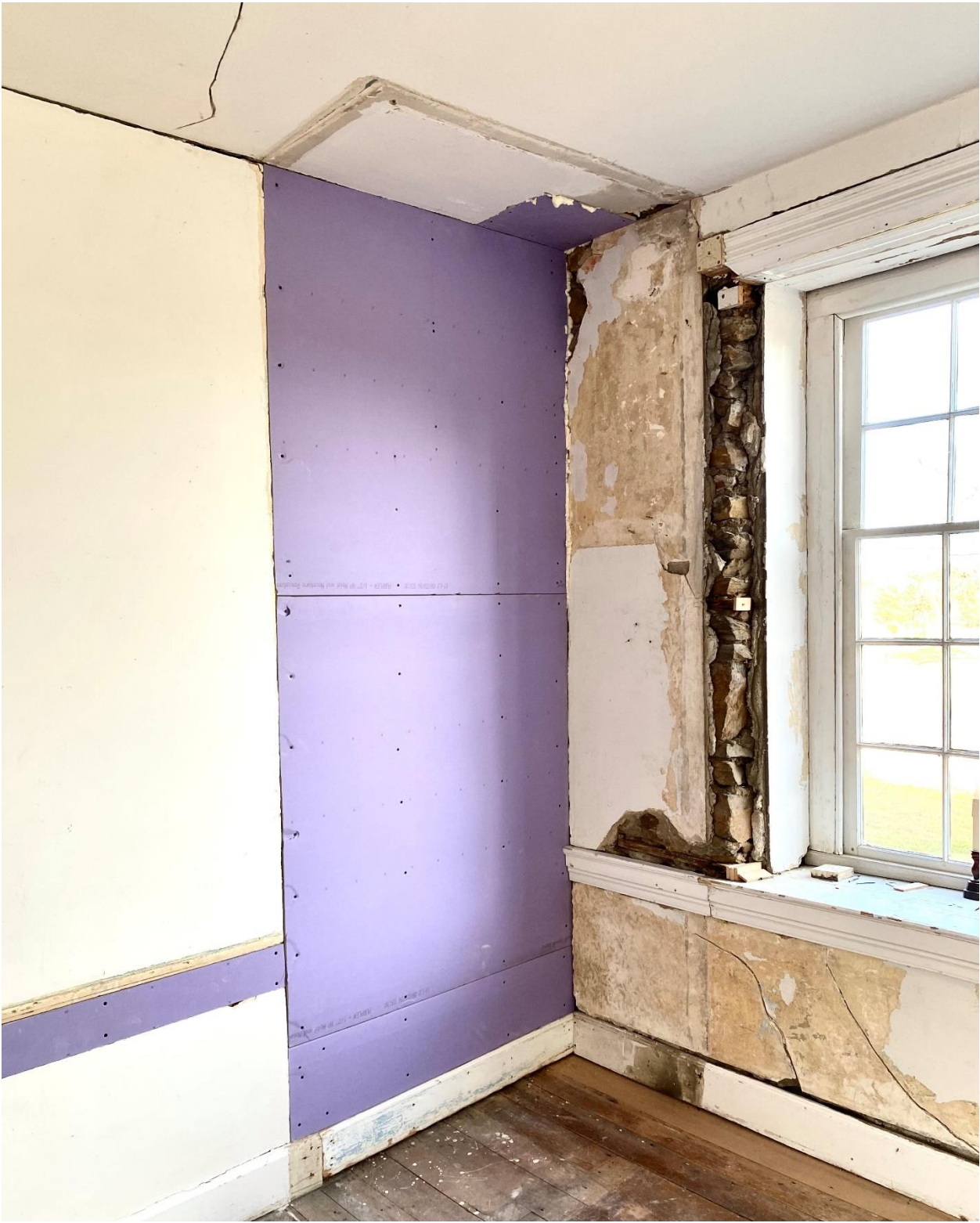
Front closet door opening infill "AFTER"
