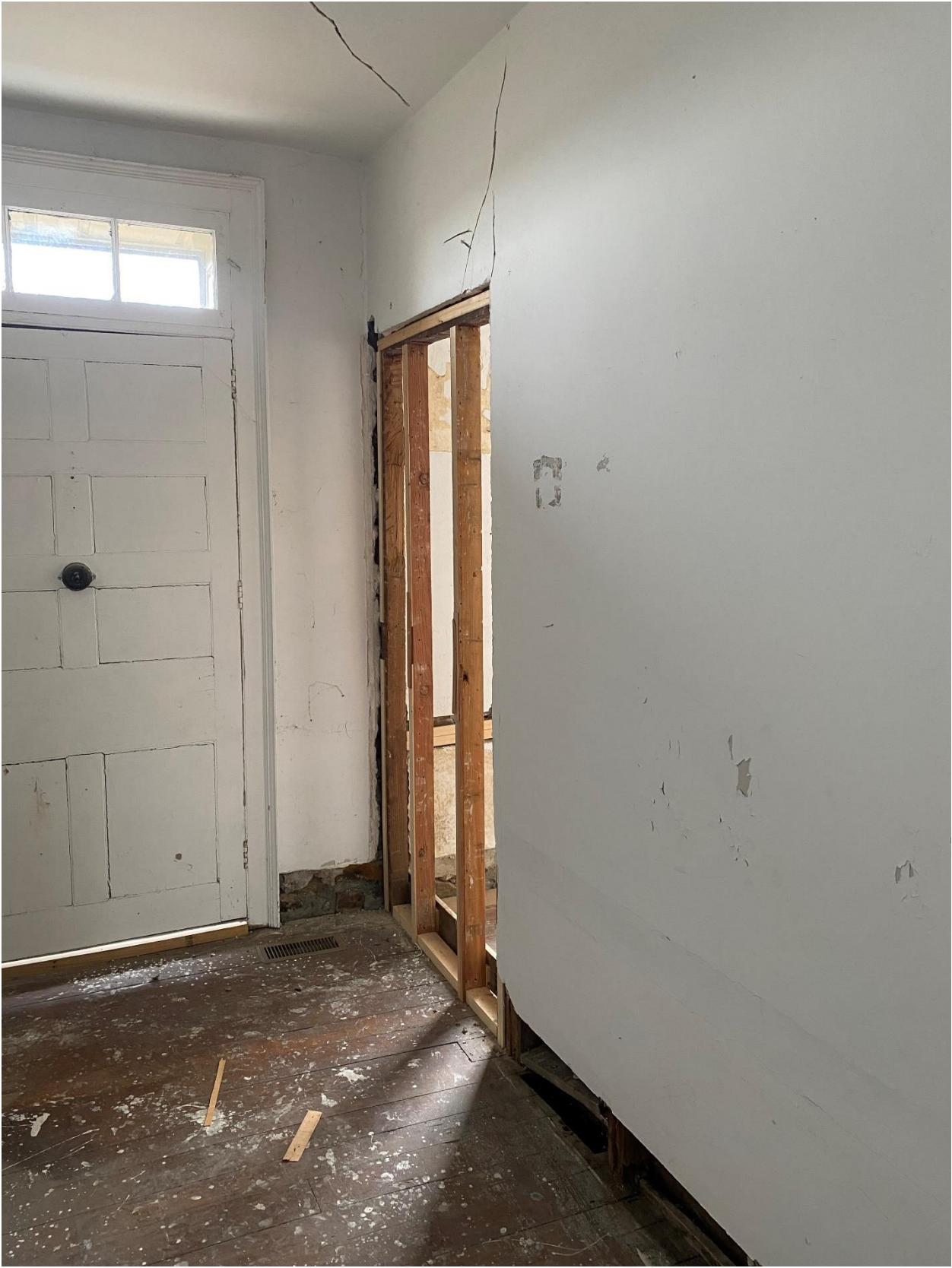
Front stair hall "BEFORE"
