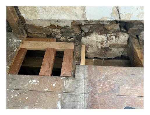
The flooring joints were staggered to give a more pleasing appearance and disguise the repair. Wood with similar grain was chosen. Once sanded and finished the area should blend well.
