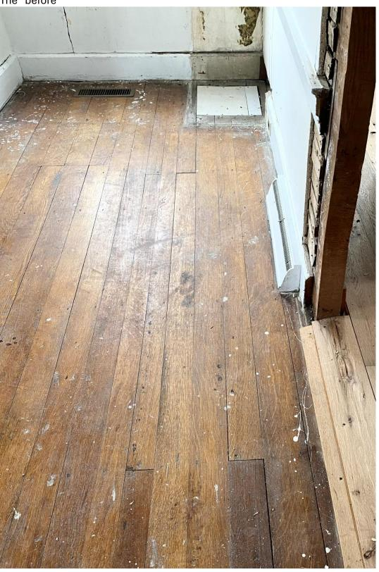
The baseboards had to be carefully removed to be able to get the flooring boards out and refit.
