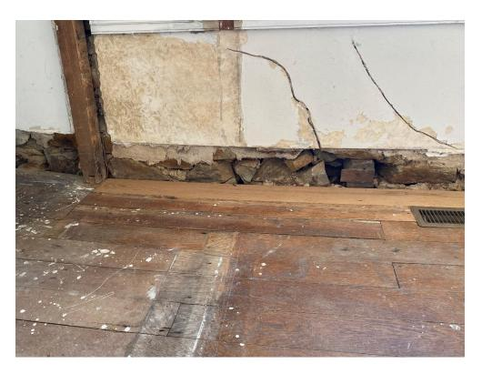
The floor in the opposite corner was also repaired. There were several duct holes that had to be removed.
