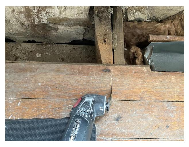
Support blocking had to be installed to carry the flooring where the former doorway and air ducts were once were located.
