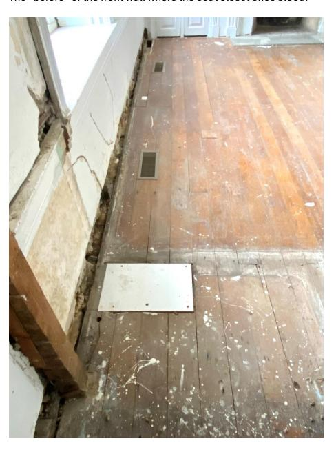
The "after" in the same location using some original boards and some "new" antique white oak flooring with similar grain. The wall infill in the former doorway will cover the joints in the floor that all line up.
